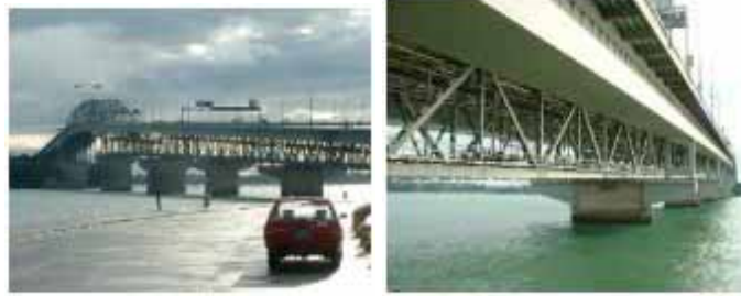
Figure 3 - A Thermal Spayed Auckland Harbour Bridge, New Zealand 3
